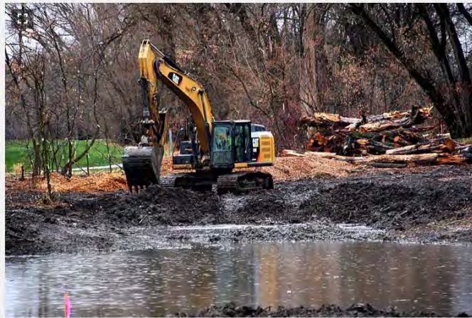
A trackhoe excavates a trench where the Logan River will soon be rerouted between the Logan River Golf Course and Rendezvous Park.
